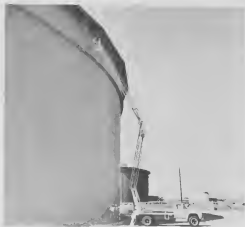
Two men of the Equipment Inspection Section are shown here aloft the 70-ft. articulated boom of the new giraffe truck at Tank 914.
